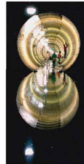
Terminated Texas tunnel. The SSC was abandoned after about 25% of the tunnel for the 87-kilometer-circumference large collider ring had been bored.
