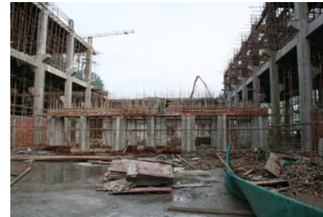
Shear wall in laser hall
